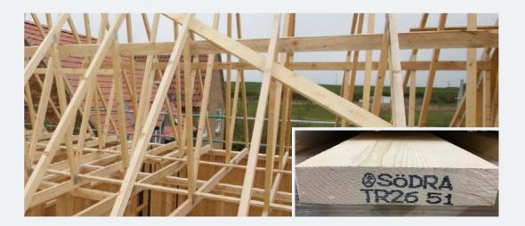
Södra has a long history of supplying machine strength graded TR26 softwood to roof truss and metal web joist manufacturers and stock an extensive range of high quality TR26 graded timber to meet the needs of our customers.
